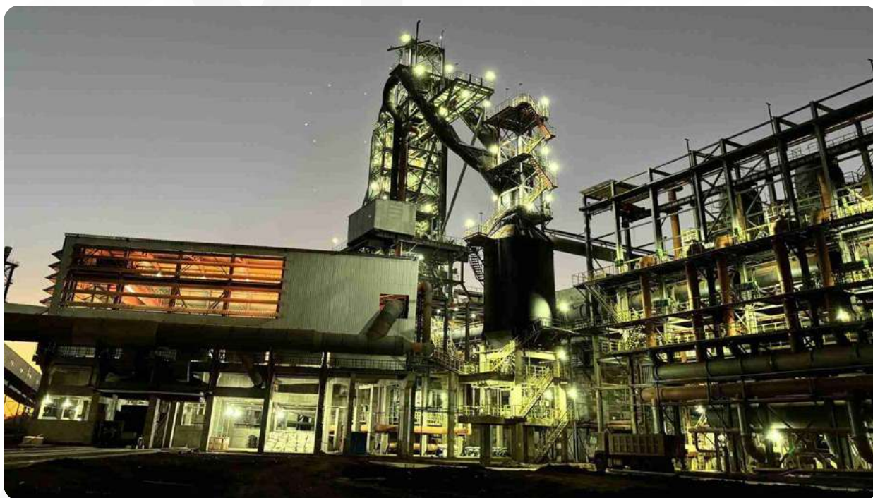
Dinson iron and Steel Company (DISCO STEEL), Manhize
